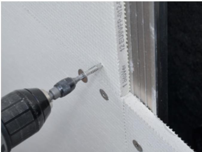
**Left:** The StoVentec R carrier board is made of 96% recycled expanded glass granulate and reinforced on both sides with glass fibre mesh for superior impact resistance.
