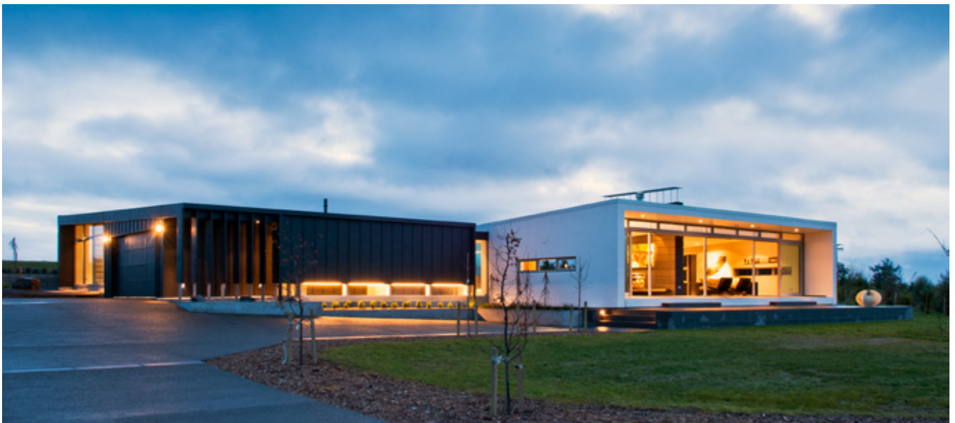
Martinborough House Architect: DesignGroup Stapleton Elliott
