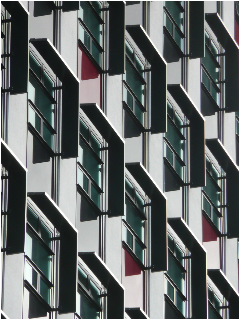
Figure 1 – External façade shading detail, East façade. Photograph: Guy Marriage
